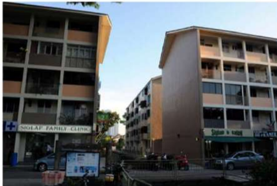
Blocks 1, 2 and 3 in East Coast Road. These blocks are about 48 years old, and there are 82 households in total. In the Selective En bloc Redevelopment Scheme (Sers), residents are compensated for their existing homes and given discounts on brand new flats. PHOTO: ST FILE
